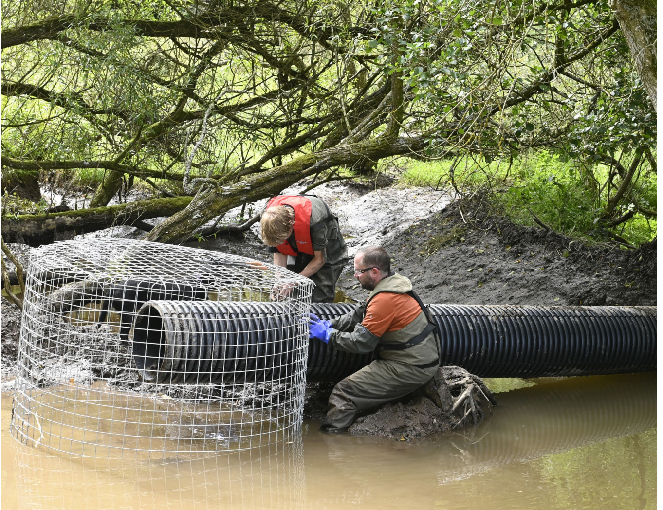
Installation of a beaver deceiver pipe at Gelly Burn, Tayside.
