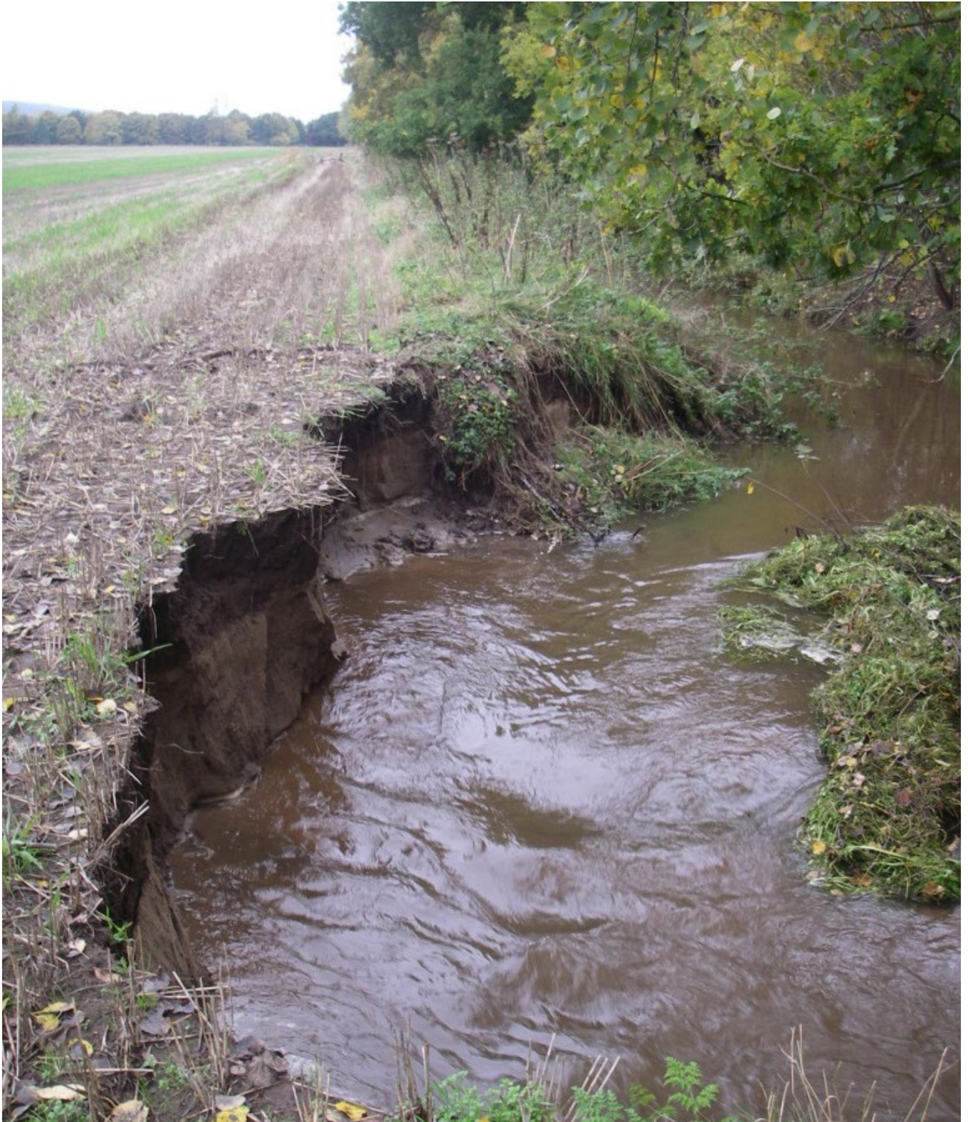
Bank erosion at a Tayside farm following diversion of water flow around a beaver dam.
