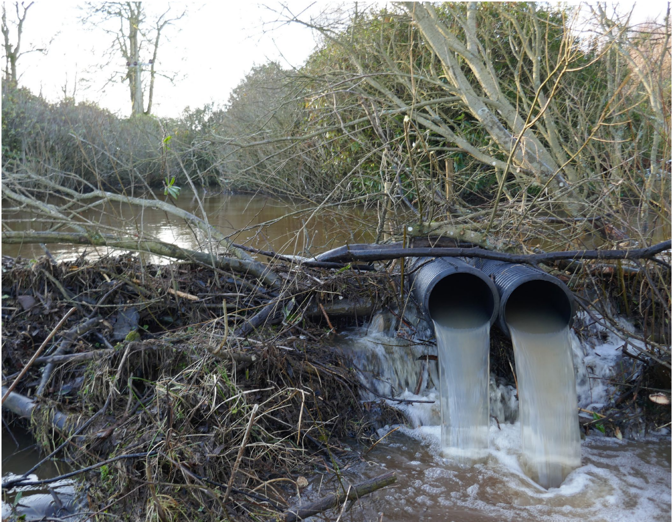
Flow device pipe installed in a beaver dam at Forfar, Tayside.
